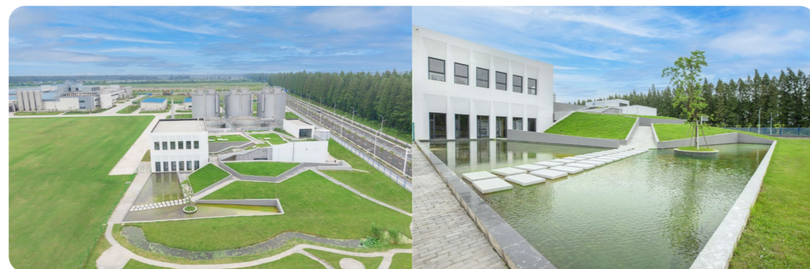
Sewage treatment station of Mengniu Wuhan Factory
